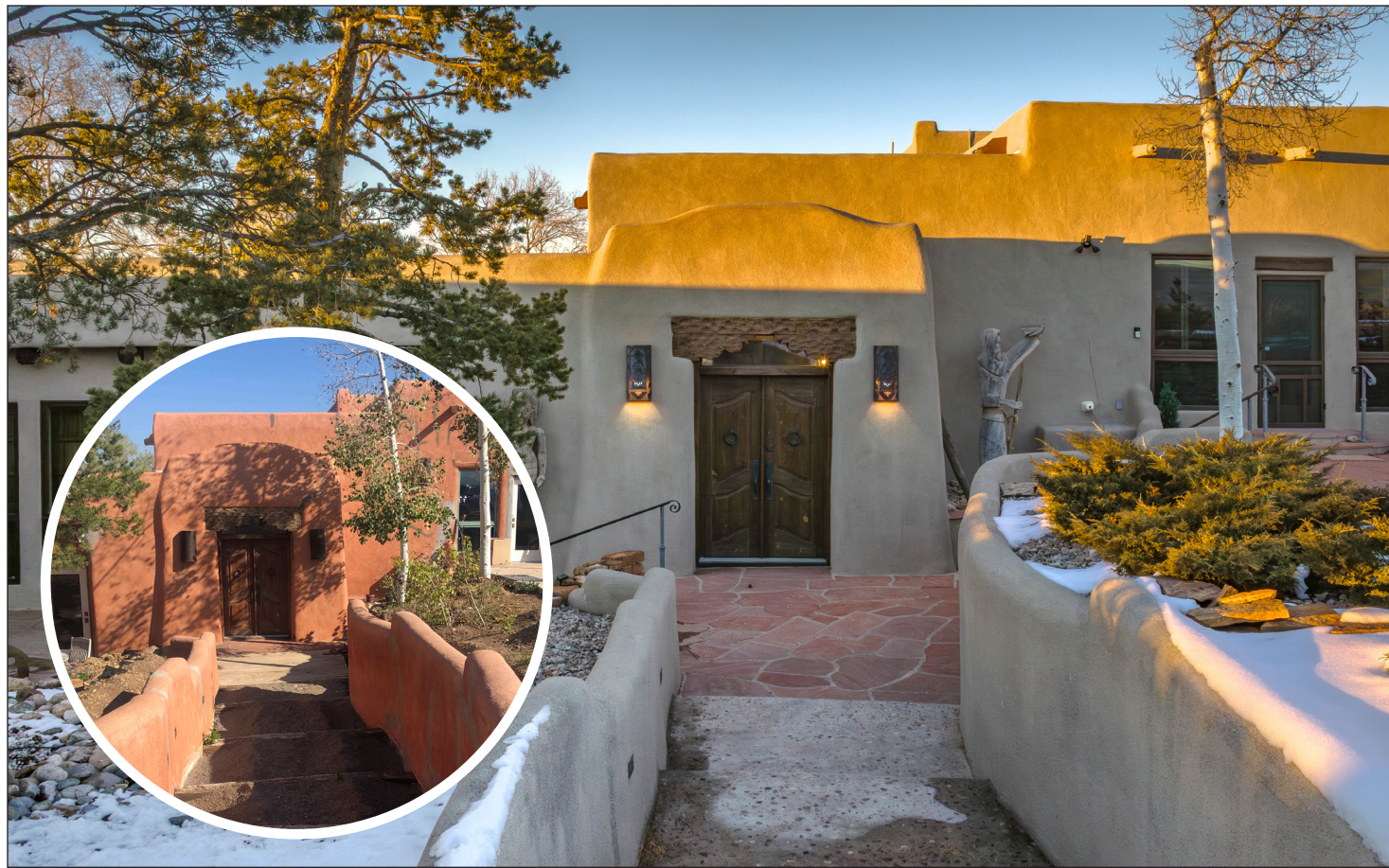
Before/After of the main house
